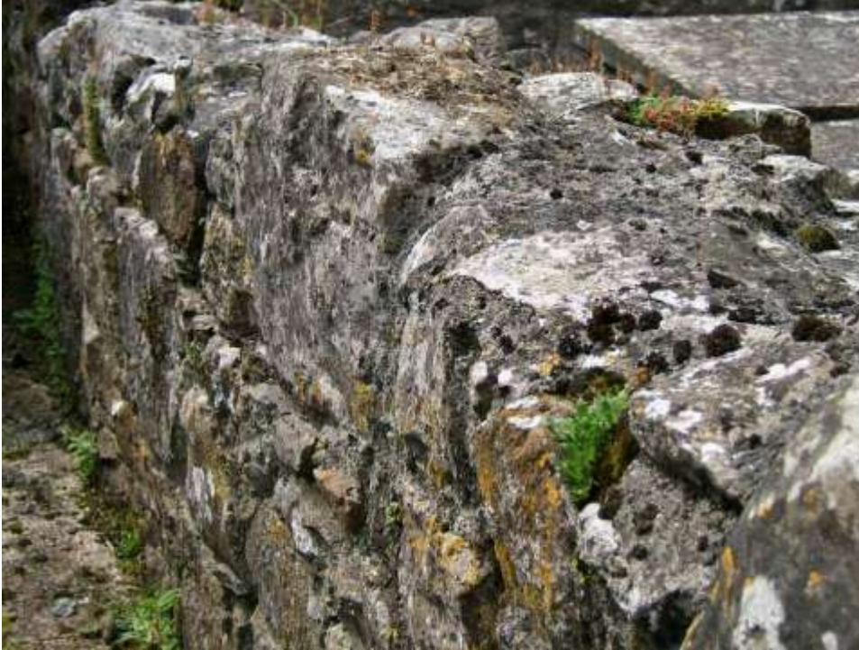
Plate 8. Biological growth on wall, Clonmacnoise (Photo C Daly 2009)
