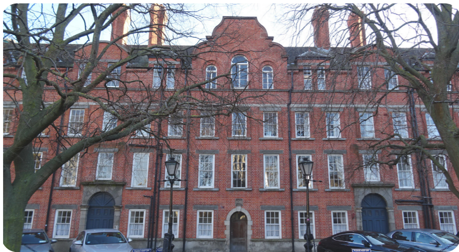
West elevation prior to the Conservation Works.
