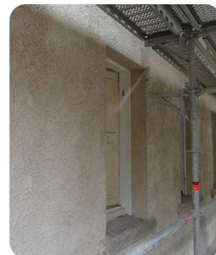
Removal of the cementitious render and new insulated external render on the east-elevation.
