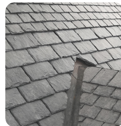
New Valentia slates to the roof.
