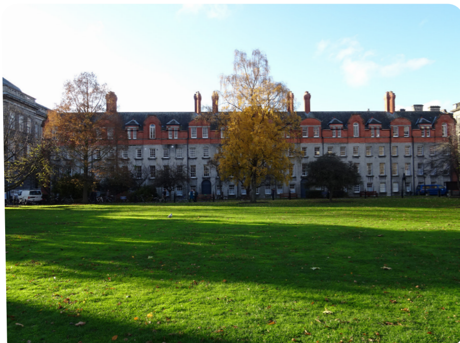
View of east elevation and New Square prior to the Conservation Works.
