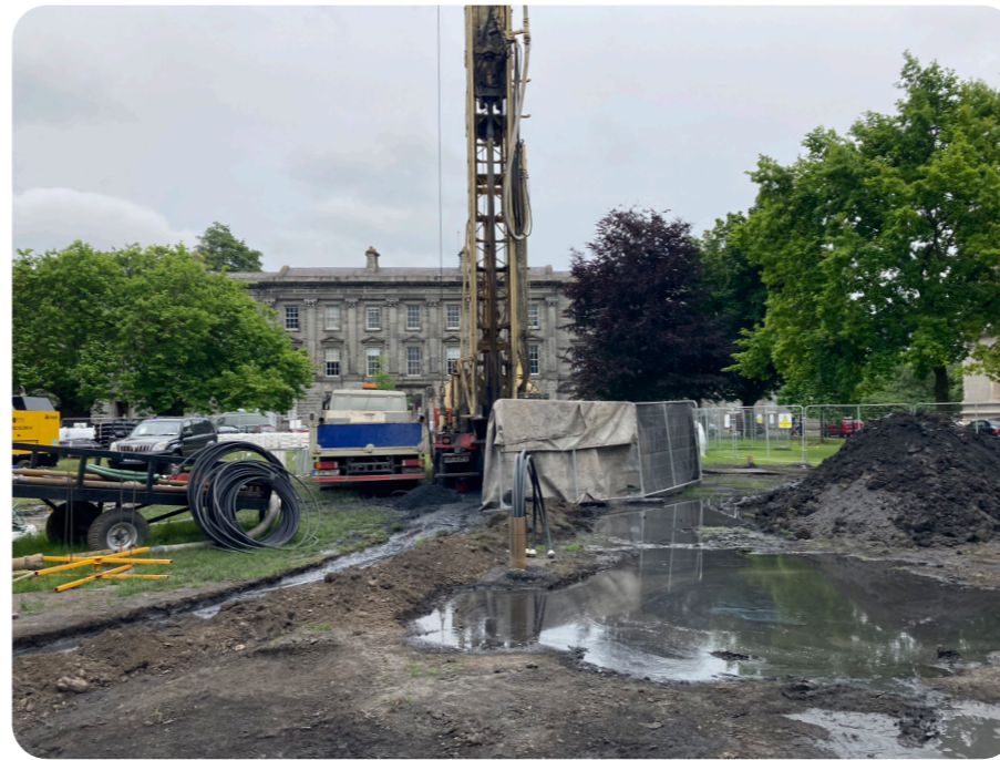
Installation of the ground collector system.
