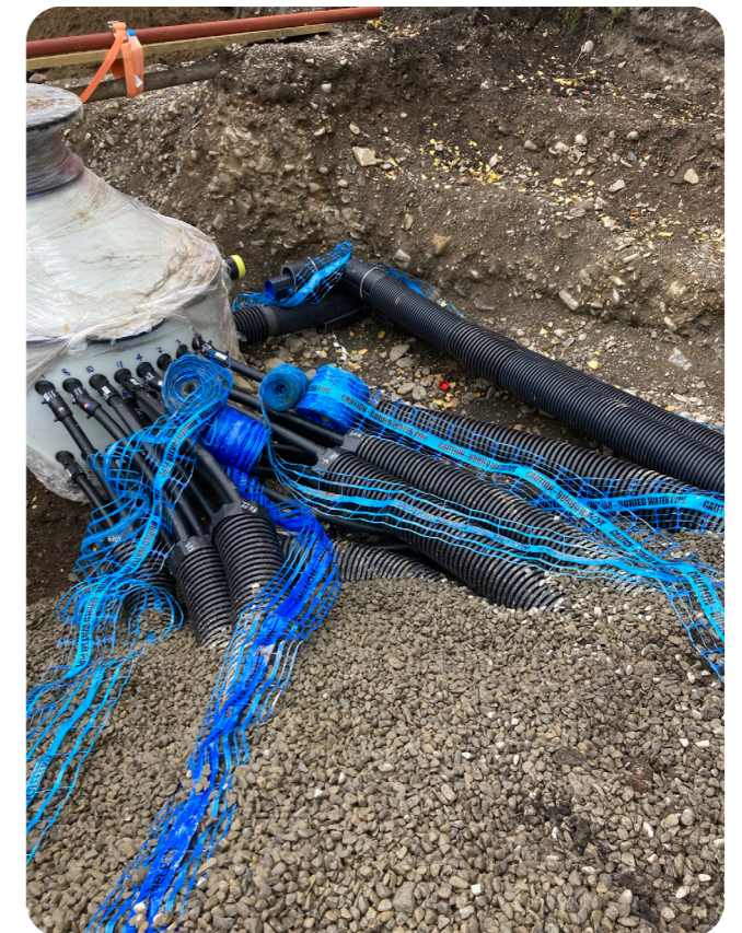
Installation of the ground collector system.
