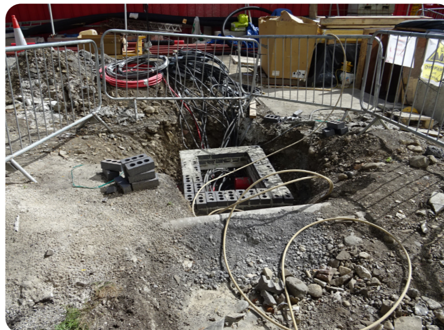
Installation of the ground collector system.
