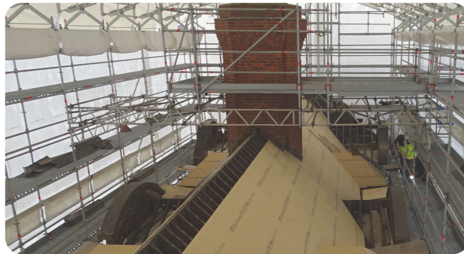
Thermal upgrade works to the roof.
