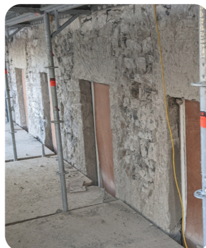
Removal of the cementitious render and new insulated external render on the east-elevation.
