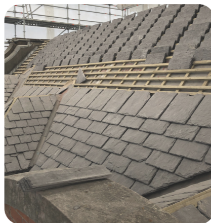
New Valentia slates to the roof.
