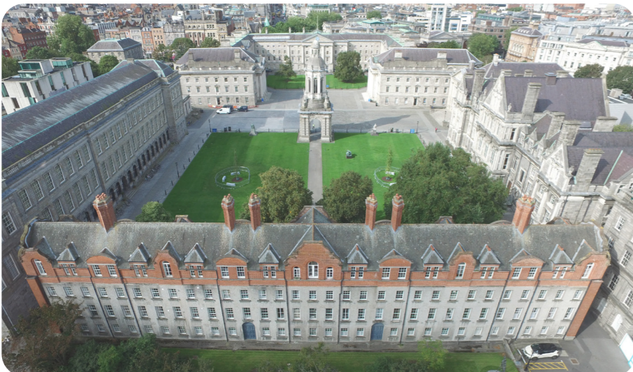
Aerial view of east elevation prior to the Conservation Works.
