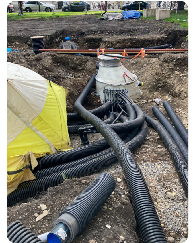
Installation of the ground collector system.
